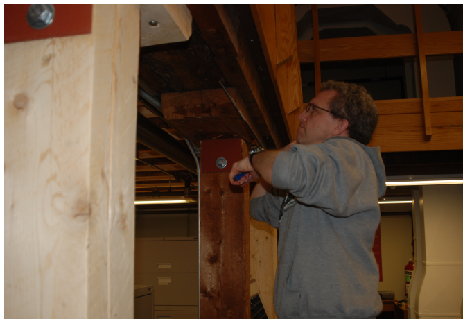
Figure 1: Coring one of the ceiling beams in the ground floor warehouse.
