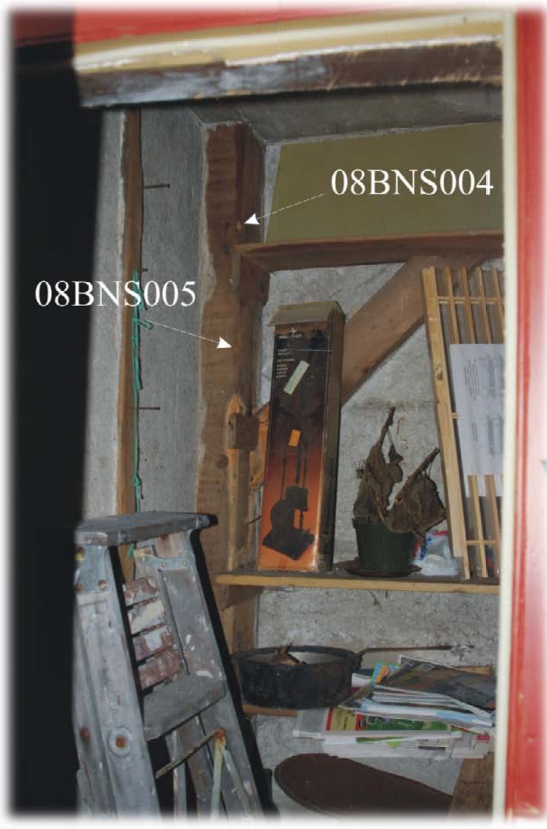
Figure 5. Samples 08BNS004/005 in the old kitchen wood closet next to the fireplace, both cores were taken from the same beam.
