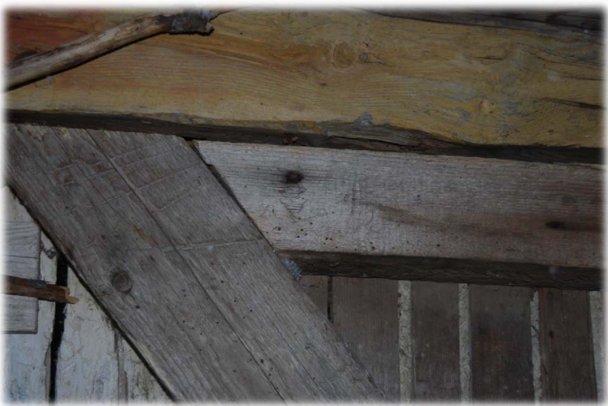
Figure 10. Photo of potentially recycled wood. The diagonal beam has roman numerals on it that do not match to either of the beams it is attached. Roman numerals are typically found on early post and beam structures.
